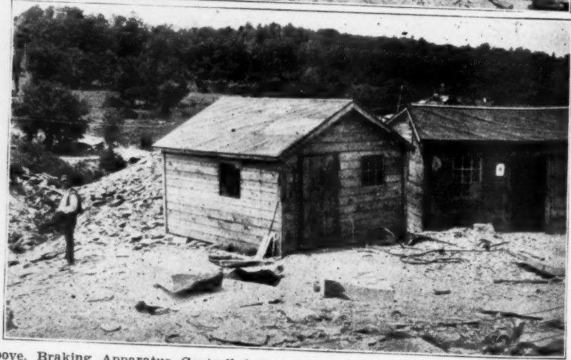
Above, Braking Apparatus Controlled from Motion House. Middle, Outdoor Transformer Bank. Below, Trimming and Splitting Houses
